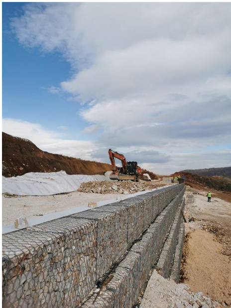
Photo 7: Section 2 Gabion Wall Works
