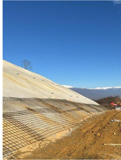
Photo 8: Section 2 Slope Protection Operations
