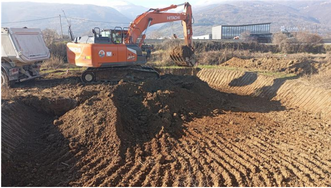
Photo 9: Section 1 Box Culvert Excavation
