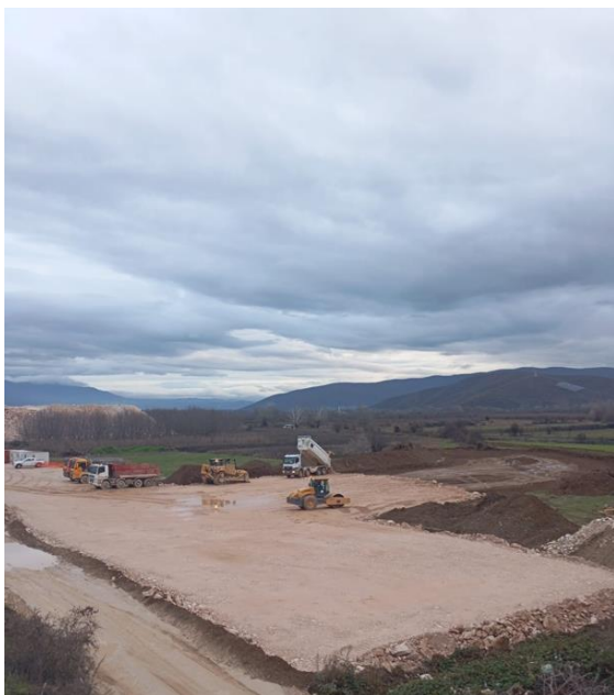
Photo 7: Section 1 Filling Operations
