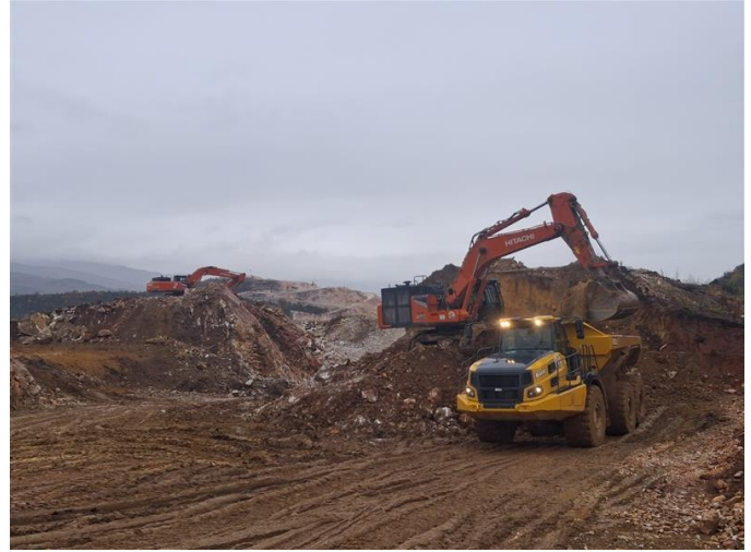
Photo 10: Section 2 Cut Section Excavation
