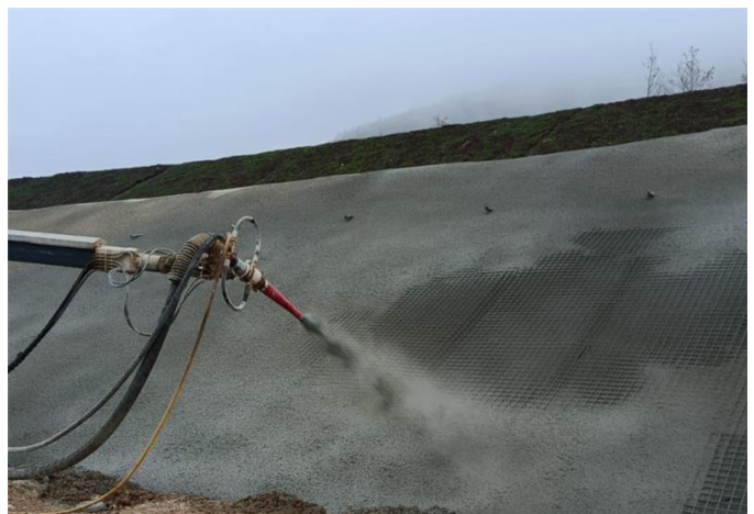
Photo 8: Section 2 Slope Protection Operations
