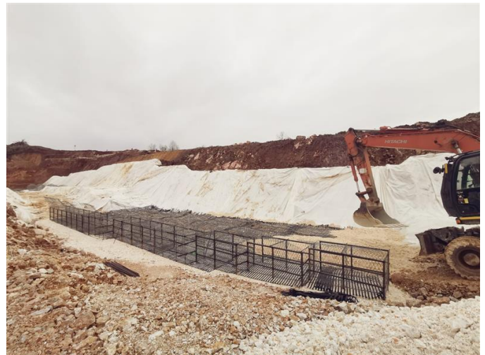
Photo 4: Section 2 Gabion Wall Works
