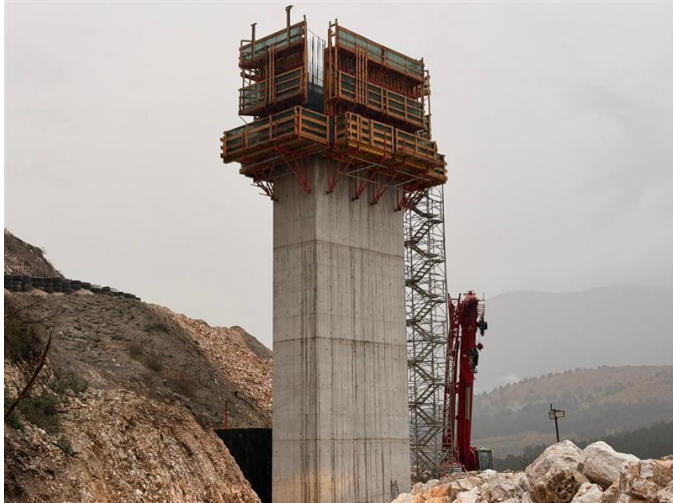
Photo 5: Section 2 B0080 Bridge Pier Elevation
