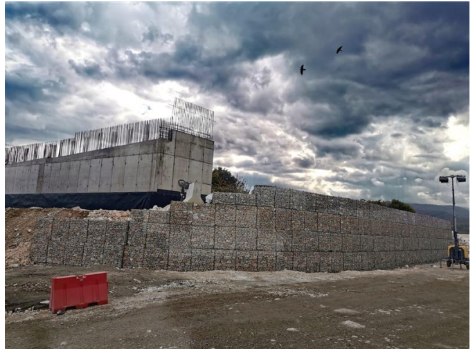
Photo 4: Section 2 Gabion Wall Works
