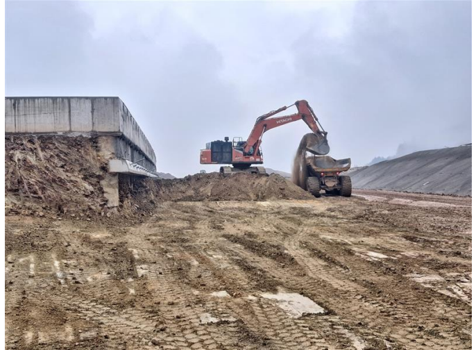
Photo 10: Section 2 Cut Section Excavation
