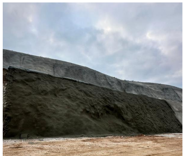
Photo 8: Section 2 Slope Protection Operations
