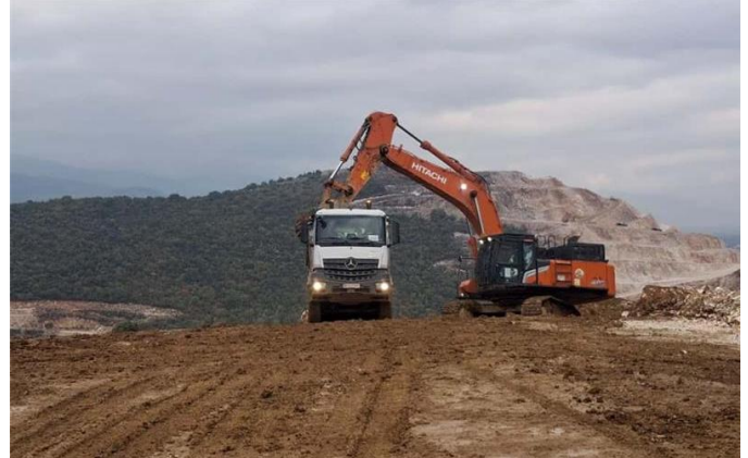
Photo 2: Section 2 Earthworks Operations
