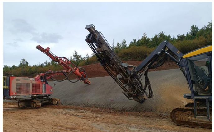
Photo 8: Section 2 Slope Protection Operations
