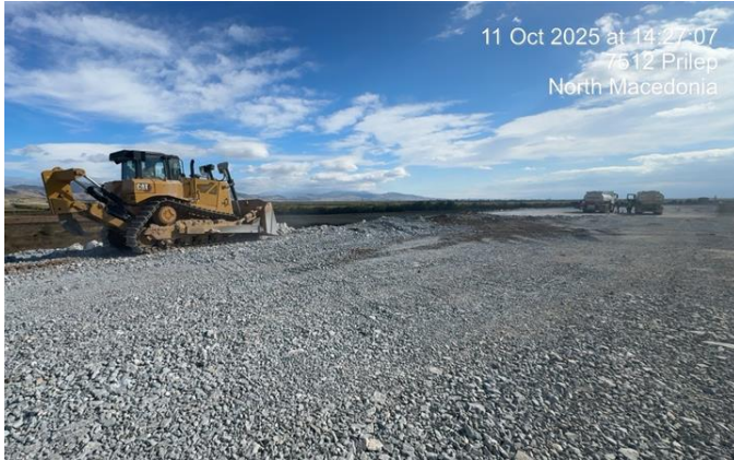
Photo 1: Section 4 Earthworks Operations
