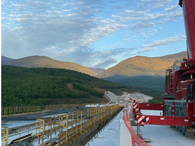
Photo 5: Section 2 B0070 Bridge Deck Slab
