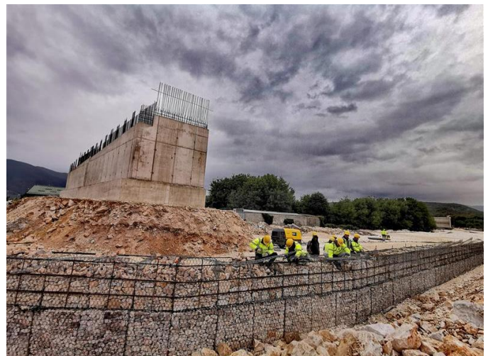
Photo 4: Section 2 Gabion Wall Works
