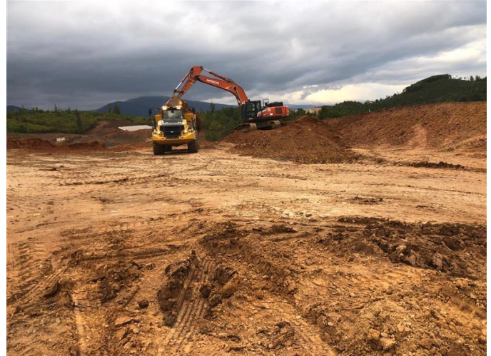
Photo 6: Section 2 Cut Section Works
