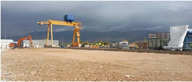
Photo 9: Section 4 Beam Yard Mobilization Works
