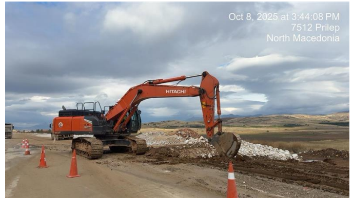
Photo 10: Section 4 Earthworks Operations
