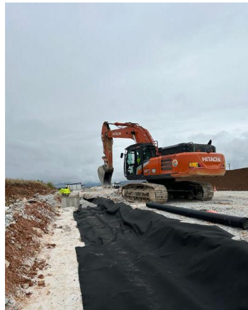
Photo 12: Section 4 Drainage Works
