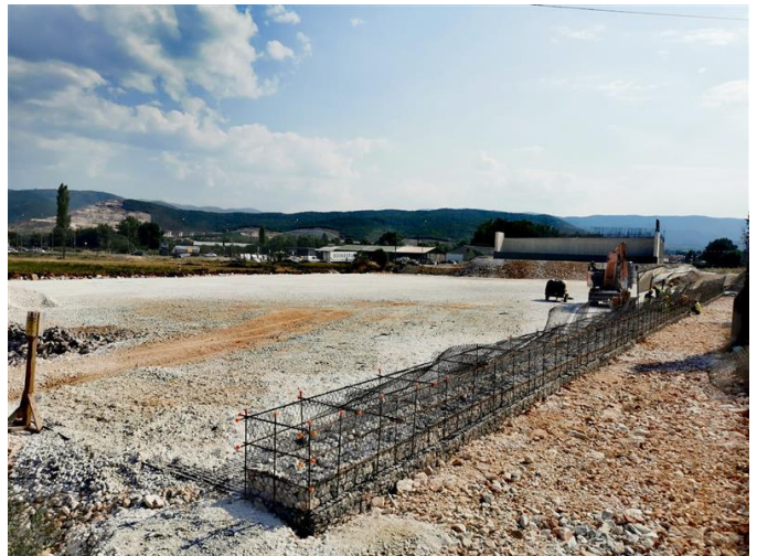
Photo 4: Section 2 Gabion Wall Works
