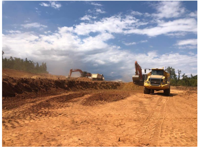
Photo 2: Section 2 Earthworks Operations
