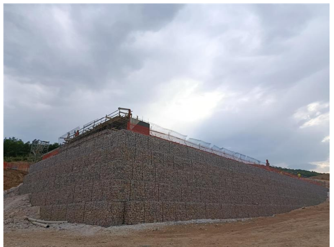
Photo 4: Section 2 Gabion Wall Works
