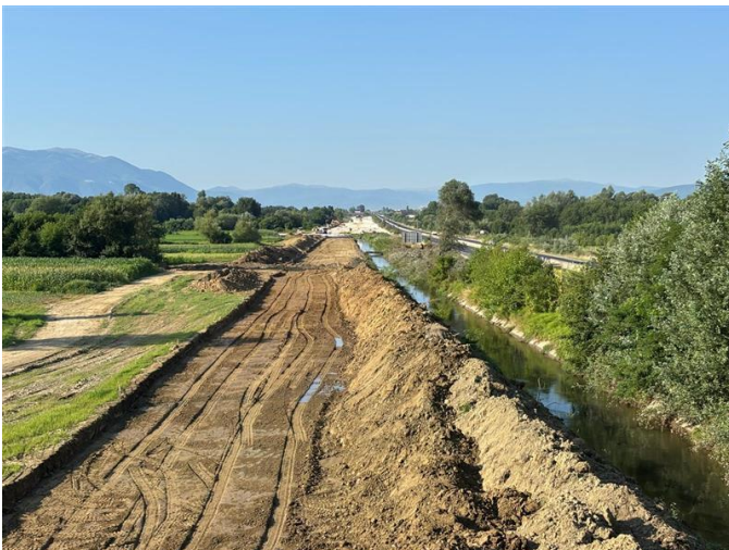
Photo 7: Section 1 Earthwork operations
