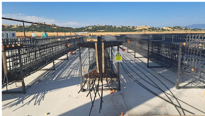
Photo 9: Section 4 Beam Yard Pretensioning and Rebar Works
