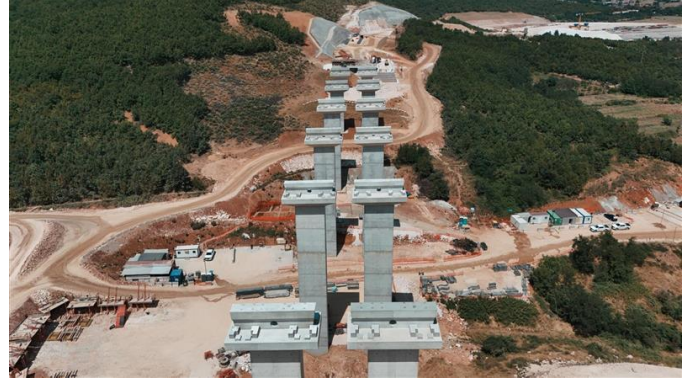
Photo 6: : Section 2 B0070 General View
