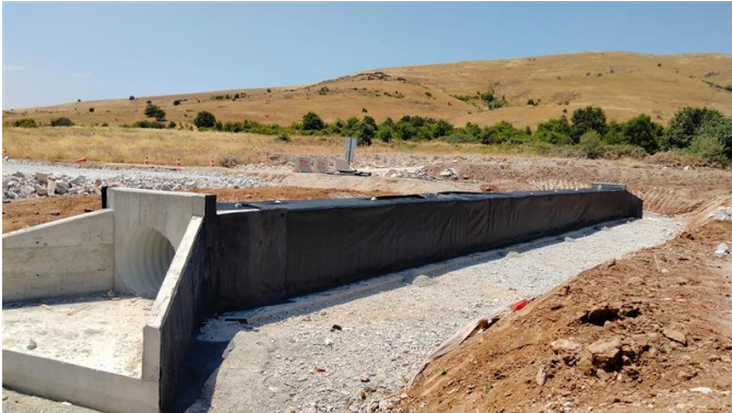
Photo 5: Section 4 Drainage Works
