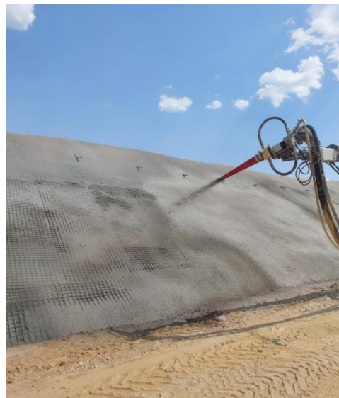
Photo 10: Section 2B Wiremesh installation and Shotcrete Operations
