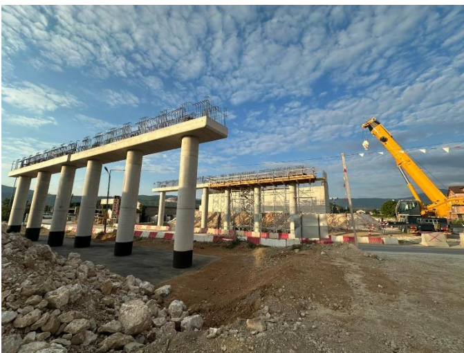
Photo 3: Section 2 B0046 General View
