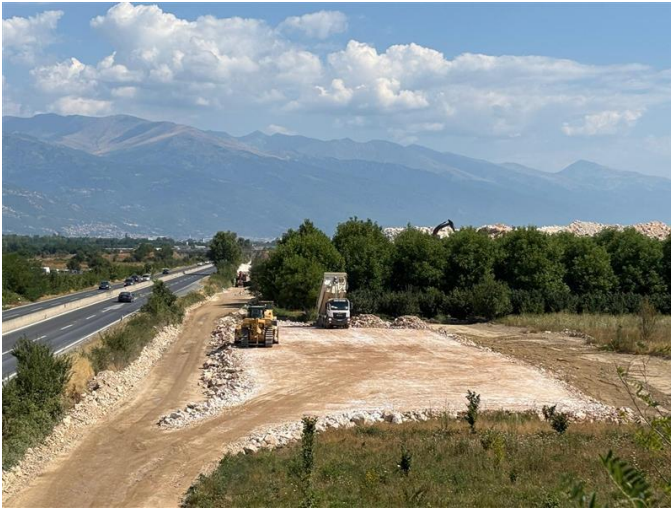
Photo 1: Section 1 Earthworks Operations
