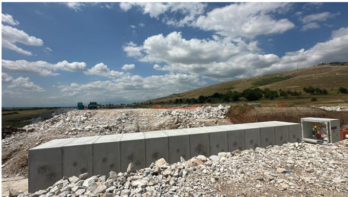
Photo 7: Section 4 - Precast Box Culvert Segment Installation
