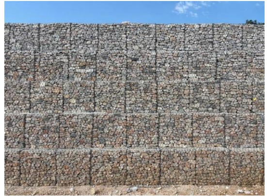
Photo 6: Section 2 Gabion Wall Works
