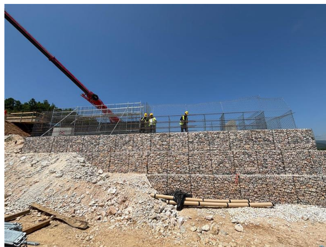
Photo 6: Section 2 Gabion Wall Works
