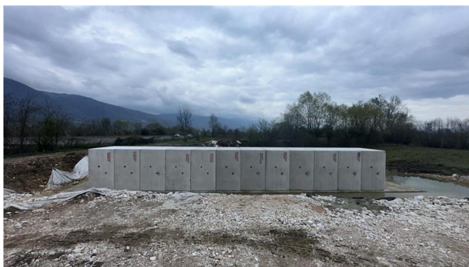
Photo 7: Section 1 Culvert Precast Segment Installation
