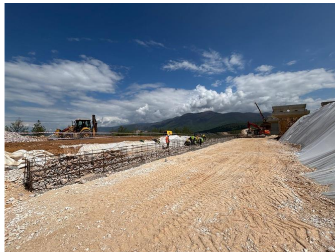
Photo 6: Section 2 Gabion Wall Works
