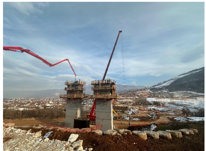
Photo 4: Section 2 B0070 Elevation Works
