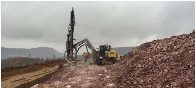
Photo 3: Section 2 Drilling and Blasting Operations
