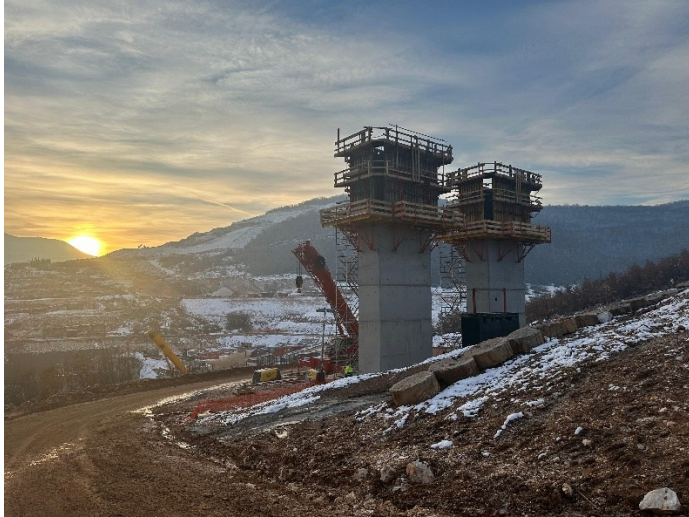
Photo 9: Section 2 Structure Works
