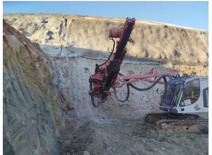
Photo 10: Section 2 Slope Protection Works
