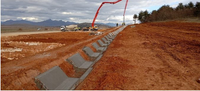
Photo 5: Section 4 Drainage Works
