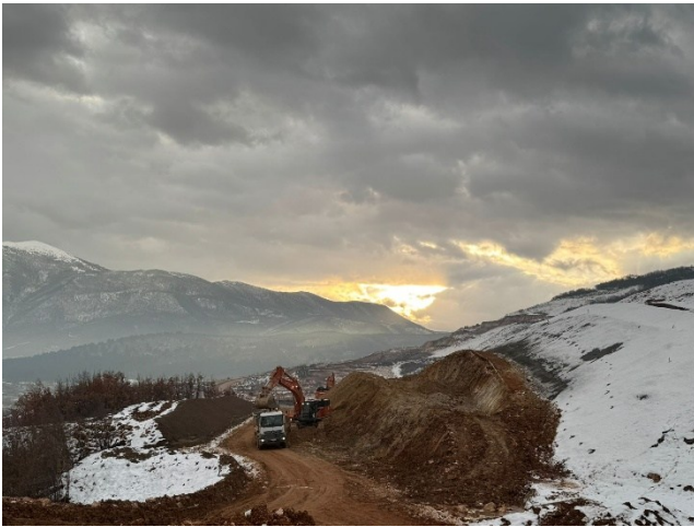
Photo 1: Section 2 Earthworks Operations
