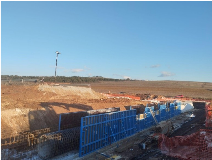
Photo 7: Section 4 Pipe Culvert Works
