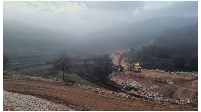
Photo 6: Section 2 Earthworks Operations
