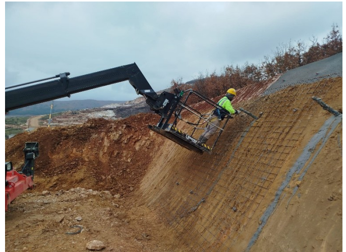
Photo 2: Section 2 Slope Protection Works
