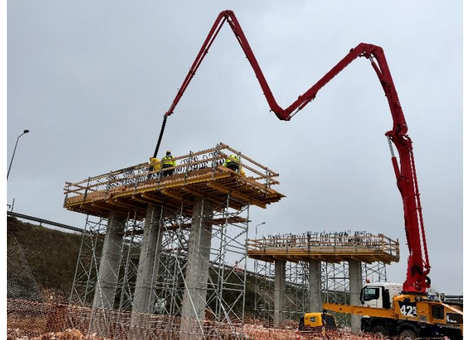
Photo 6: Section 2 Structures Operations
