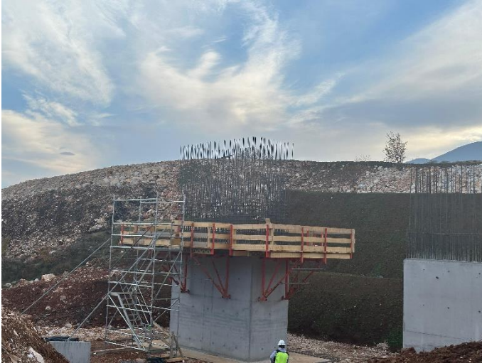
Photo 5: Section 2 Structures Operations
