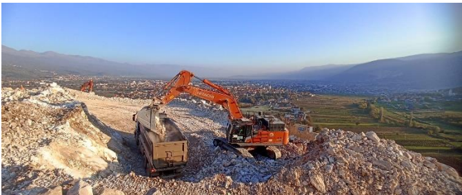
Photo 1: Section 2 Earthworks Operations
