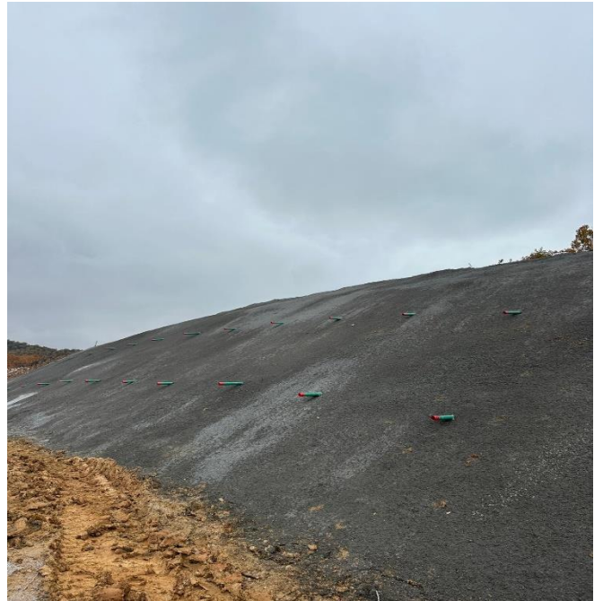
Photo 2: Section 2 Slope Protection Works
