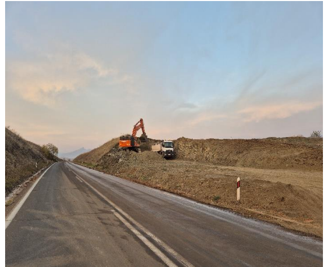
Photo 10: Section 4 Earthworks Operations
