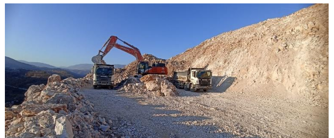
Photo 8: Section 2 Earthworks Operations
