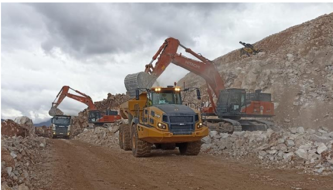
Photo 7: Section 2 Earthworks Operations
