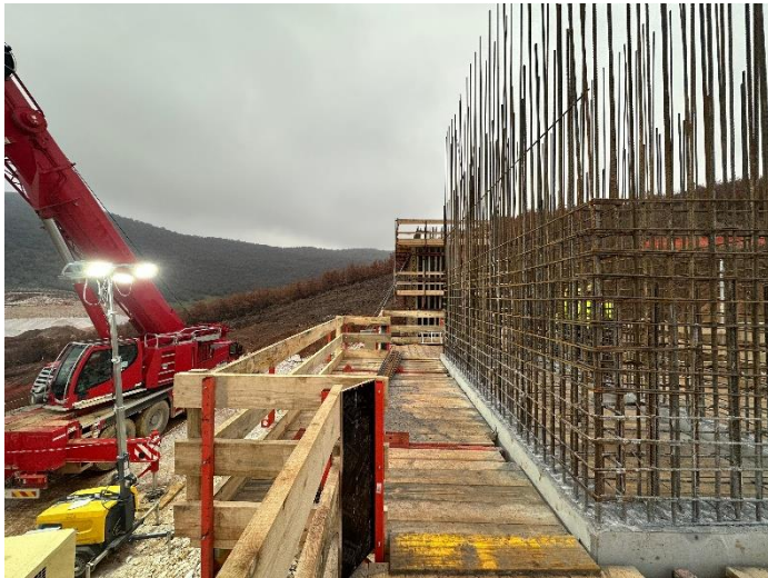
Photo 9: Section 2 Structure Works
