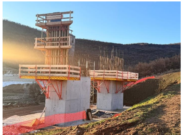
Photo 4: Section 2 B0070 Elevation Works
