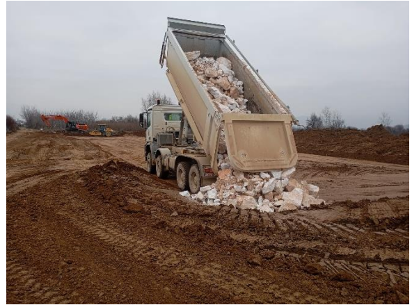
Photo 10: Section 2 Earthworks Fill Operations
