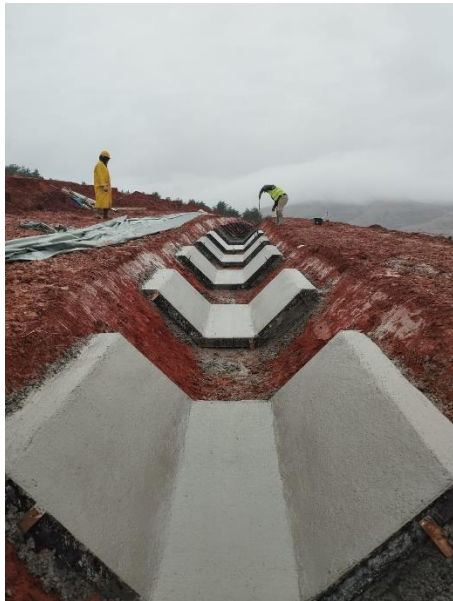
Photo 5: Section 4 Drainage Works
