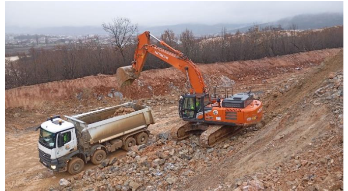
Photo 6: Section 2 Earthworks Operations
