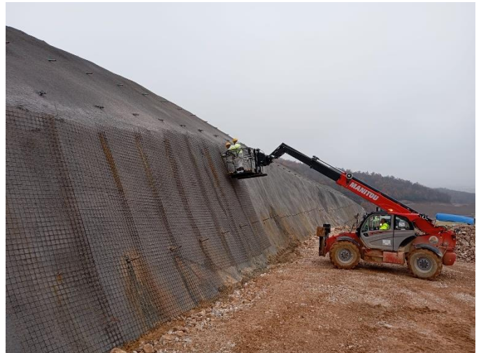
Photo 2: Section 2 Slope Protection Works
