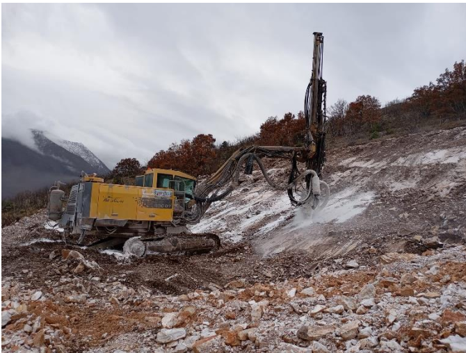
Photo 3: Section 2 Drilling and Blasting Operations
