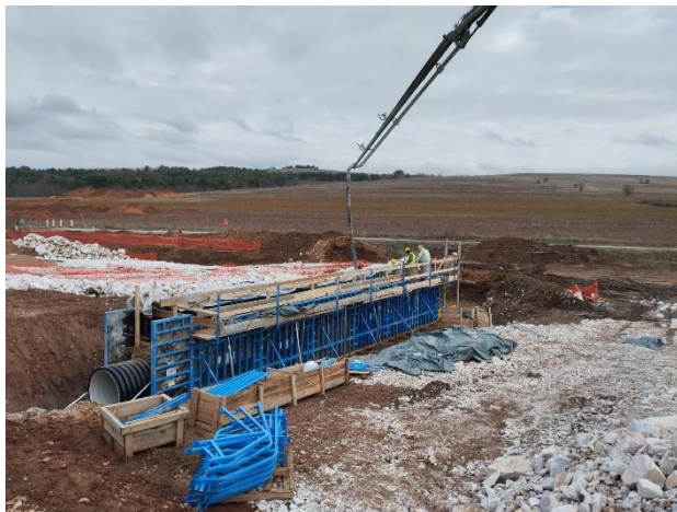
Photo 7: Section 2 Pipe Culvert Works
