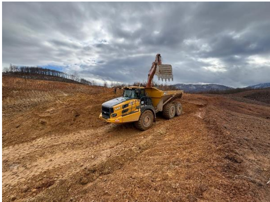
Photo 1: Section 2 Earthworks Operations
