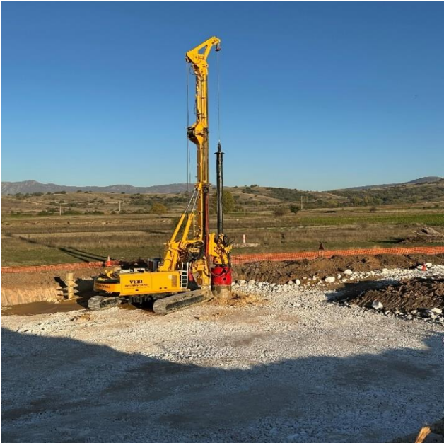
Photo 5: Section 4 Piling Operations
