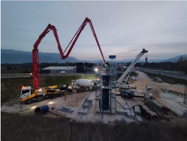
Photo 9: Section 1 Elevation Concrete Works
