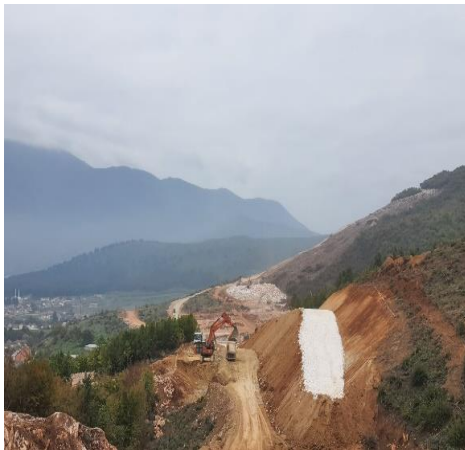
Photo 3: Section 2 Earthworks Operations
