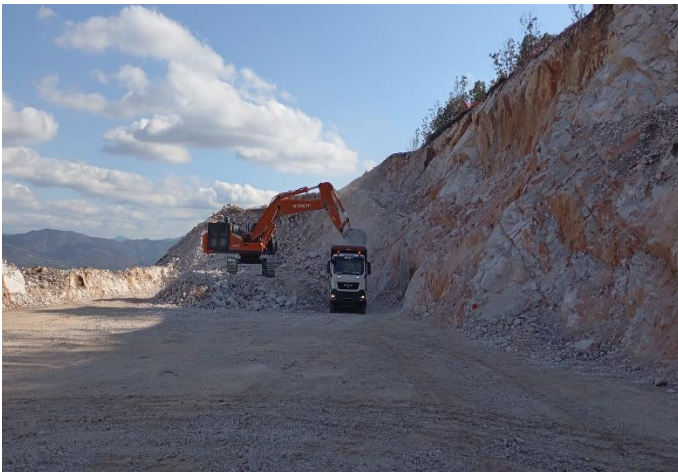
Photo 7: Section 4 Earthworks Operations
