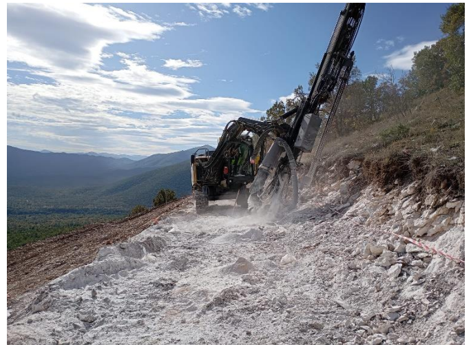
Photo 8: Section 4 Drilling Works
