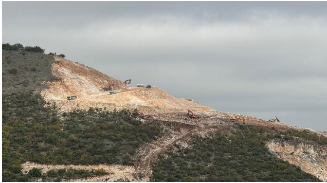
Photo 1: Section 2 Earthworks Operations
