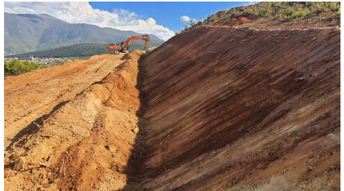
Photo 2: Section 2 Slope Protection Works
