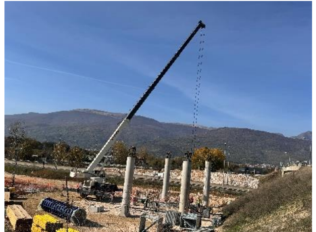
Photo 10: Section 1 Pier Elevation Works
