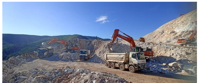
Photo 4: Section 2 Earthworks Operations
