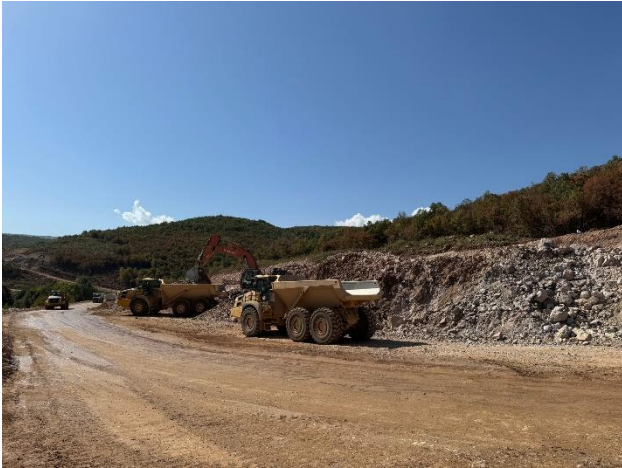
Photo 1: Section 2 Excavation Earthworks
