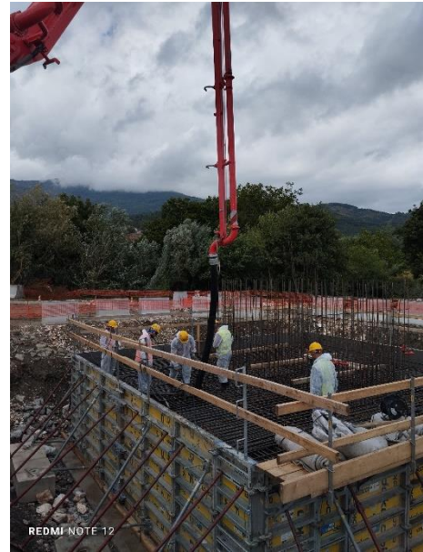
Photo 6: Section 2 Bridge Foundation Concrete Works
