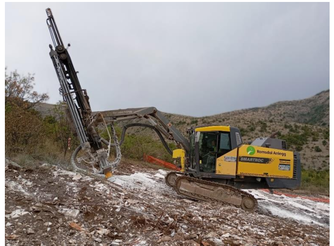
Photo 8: Section 4 Drilling Works
