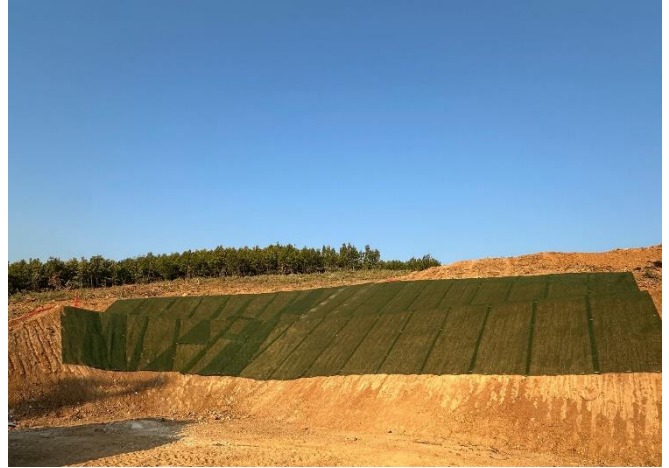
Photo 2: Section 2 Slope Protection Works
