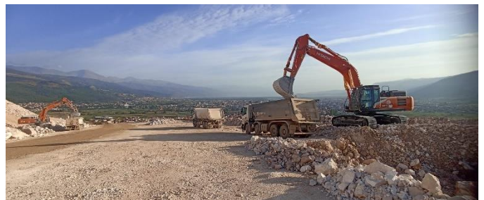
Photo 4: Section 2 Excavation Earthworks
