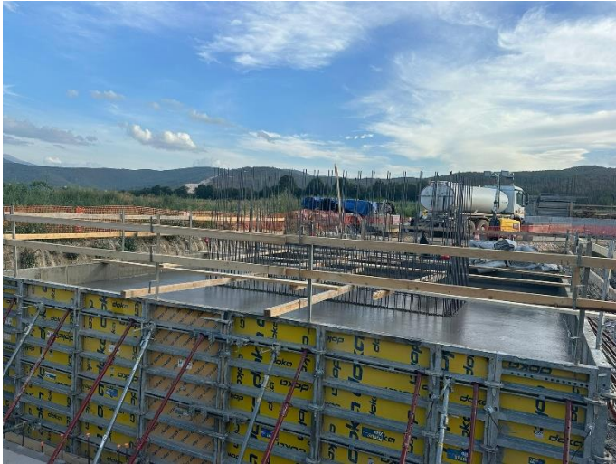
Photo 5: Section 2 Bridge Foundation Concrete Works
