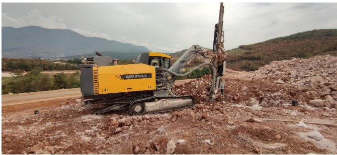
Photo 3: Section 2 Drilling Works
