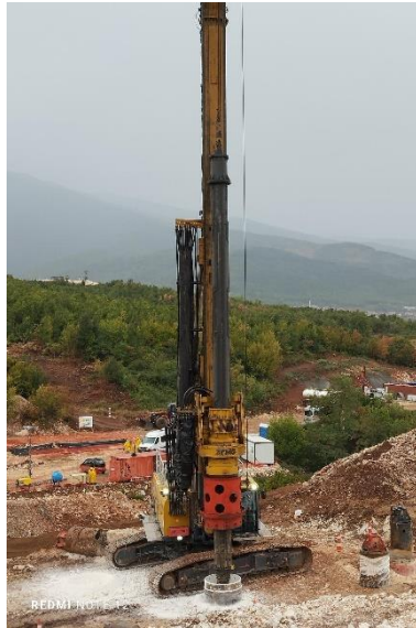
Photo 7: Section 2 B070 Piling Works
