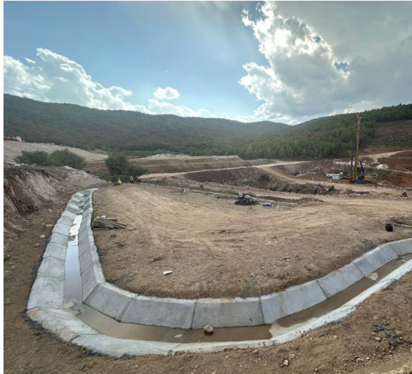
Photo 9: Section 2 Beam Yard Filling Works
