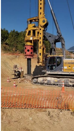
Photo 5: Section 2 B0070 Piling Works
