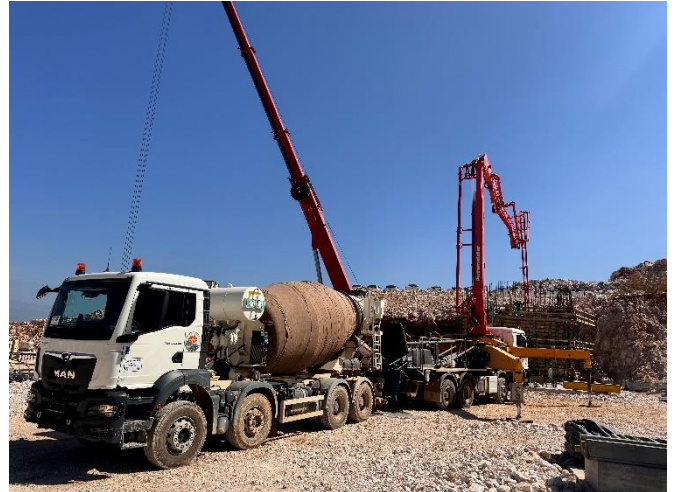
Photo 10: Section 2 Crusher Area
