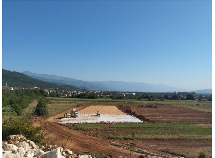
Photo 2: Section 2 Main Alignment Embankment Works
