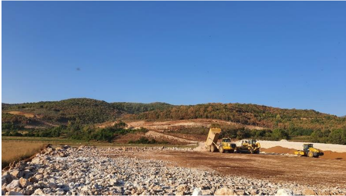
Photo 9: Section 2 Beam Yard Filling Works
