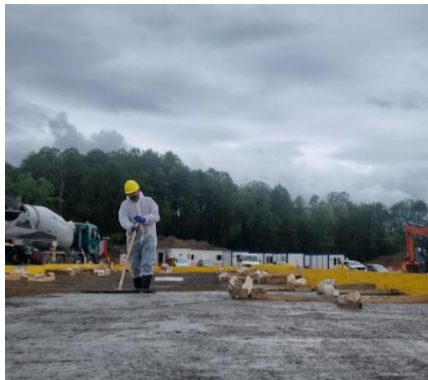
Photo 1: Section 1 Camp Area Foundation Works
