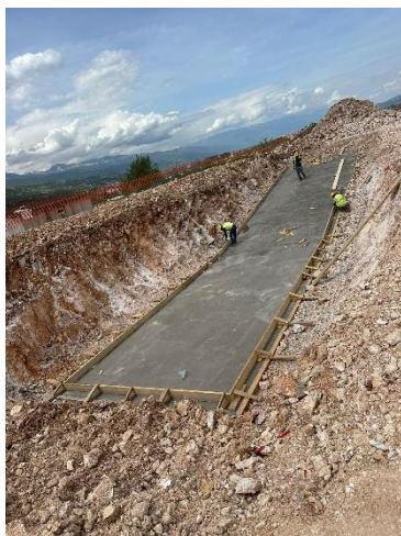
Photo 3: Section 2 Batch Plant Foundation Works
