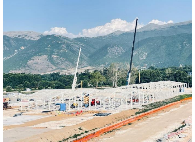
Photo 6: Section 1 Camp Construction
