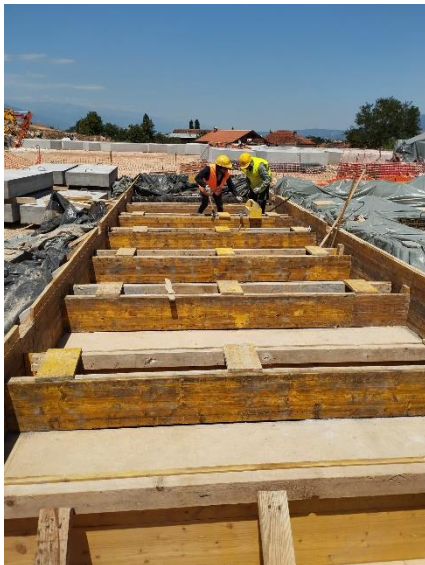
Photo 3: Section 2 Precast Yard Slab Formwork
