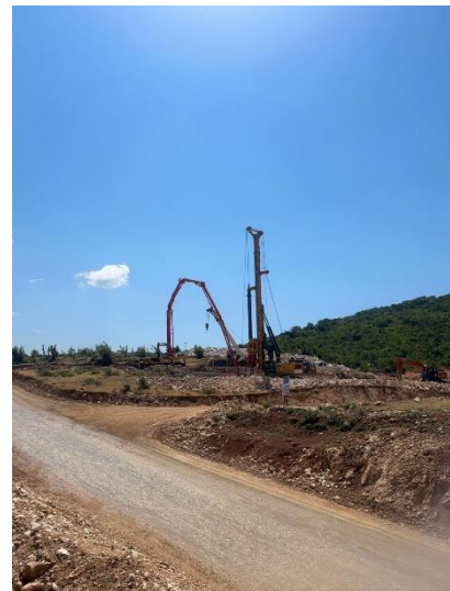
Photo 4: Section 2 B0051 Piling Operation
