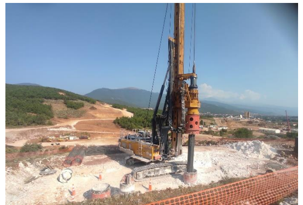
Photo 8: Section 2 - Bridge Piling
