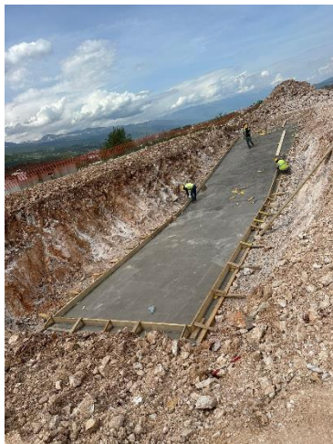
Photo 3: Section 2 Batch Plant Foundation Works
