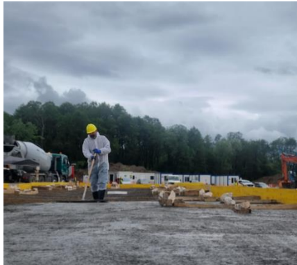
Photo 1: Section 1 Camp Area Foundation Works
