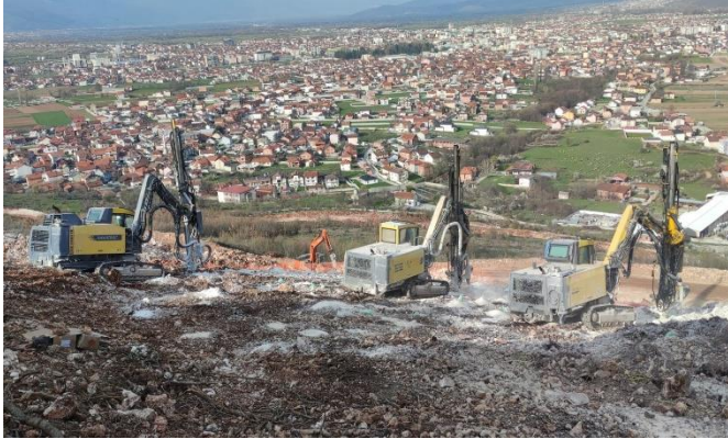
Picture 11: Section 2 - Km 7+500 - Drilling Works
