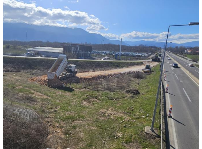
Picture 2: Section 1 Overpass 7, access road to Piling Platform
