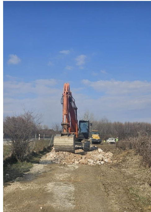
Picture 8: Section 1 LHS - Km 52+200 - Road improvement works
