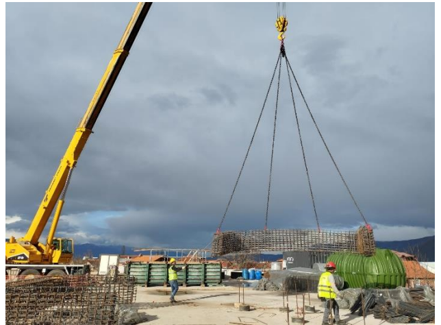
Picture 4: Section 2 - Km 6+800 - Precast Box Culvert
