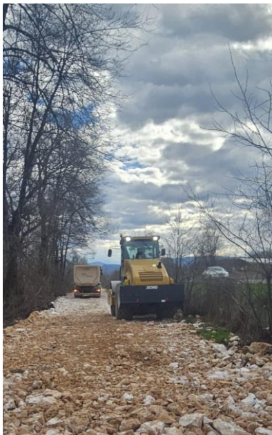
Picture 9: Section 1 - Km 51+100 - existing road improvement filling works
