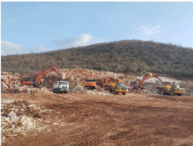
Picture 5: Section 2 - Crusher Area excavation works.
