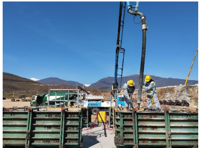
Picture 10: Section 2 - Km 6+800 Precast Yard - Segment Production
