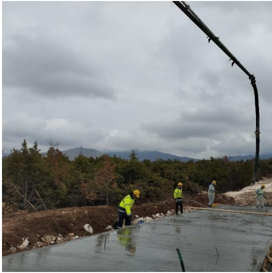
Picture 7: Section 4 Borrow pit 6 Weighbridge foundation concrete pouring
