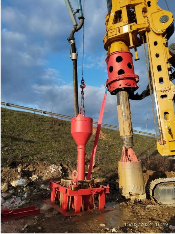
Picture 1: Section 1 - Overpass at km 49+875 - Concreting First Piling
