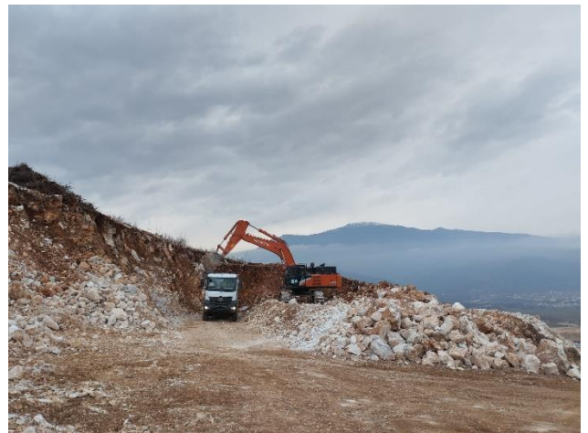
Picture 6: Section 2 - Km 7+400 excavation works
