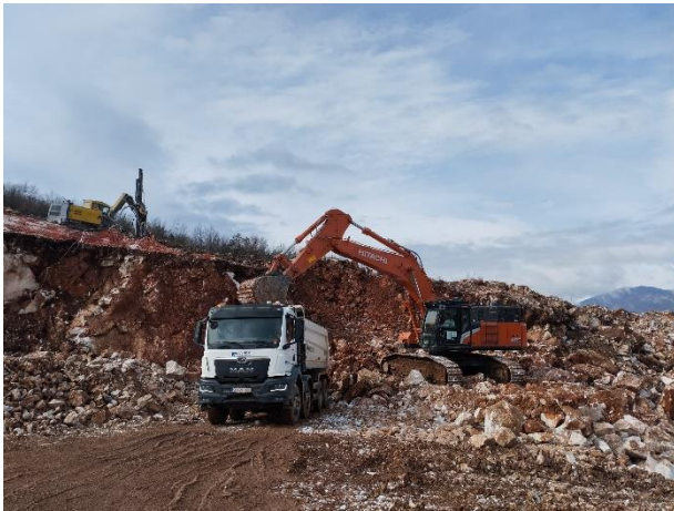
Picture 3: Section 2 - 7+400 loading and block crushing works for S1 stock area.
