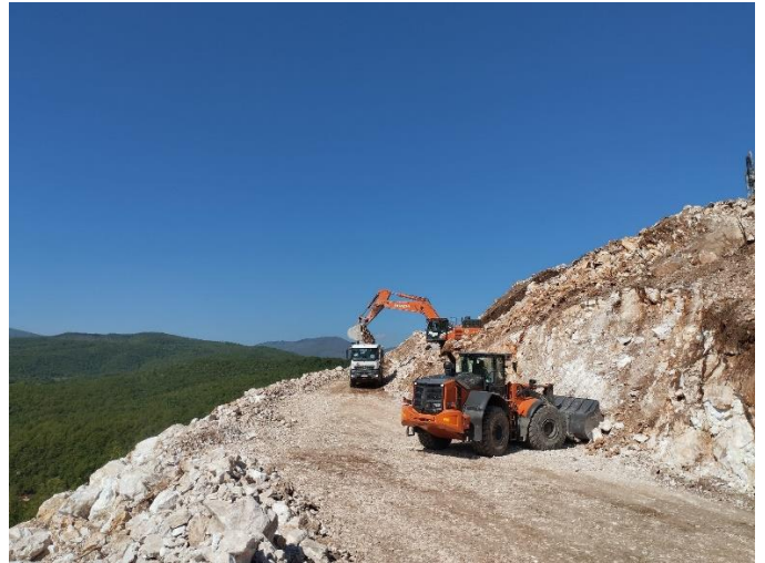
Picture 2: Section2 Km 7+600 and 7+850. Excavation and Hauling EW
