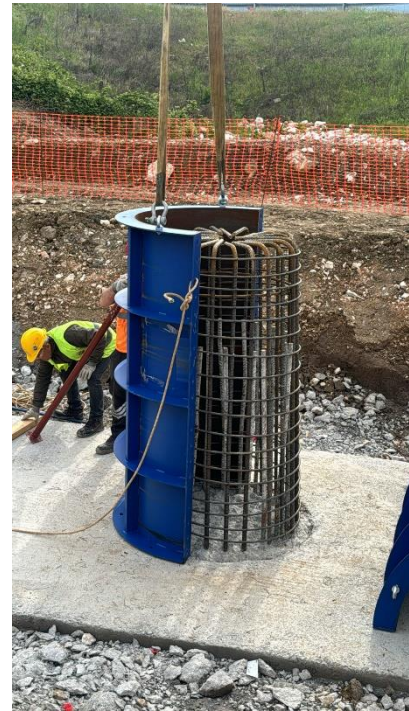
Picture 12: 49+800 Overpass-7 Formwork for PDA test of the pile
