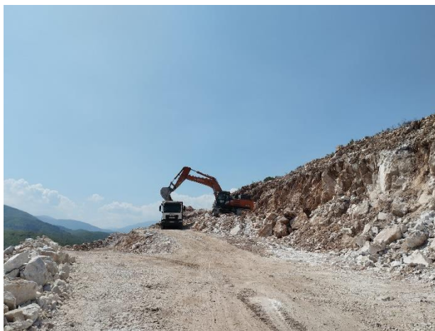
Picture 5: Section 2 - Crusher Area excavation works.
