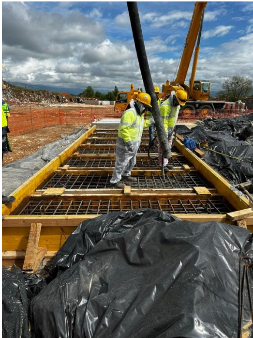
Picture 7: Precast Slab Rebar and Concrete Works
