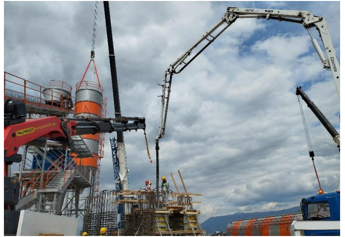
Picture 10: Section 2 - Km 6+500 - Batch Plant Area - Concrete Works
