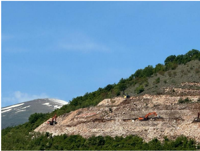
Picture 9: Section 2A Km 7+500 Earthworks Activities
