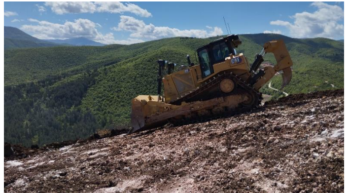
Picture 8: Section 2A Km 7+500 Earthworks Activities
