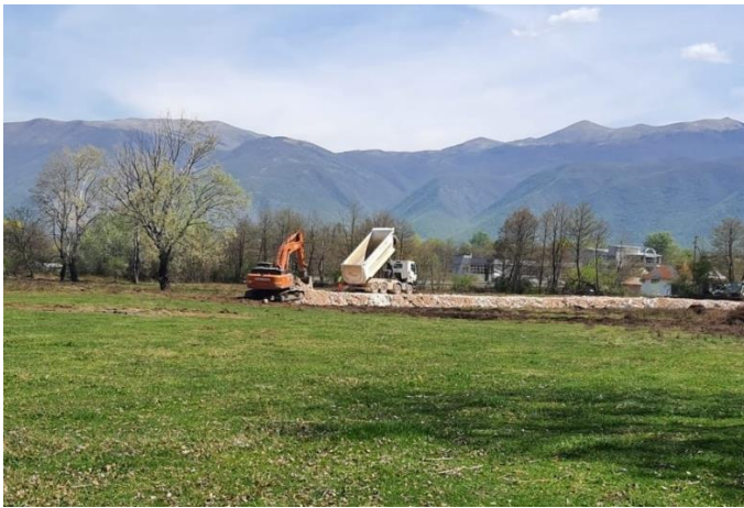
Picture 3: Clearing & Grubbing Operation at Gostivar Camp Area
