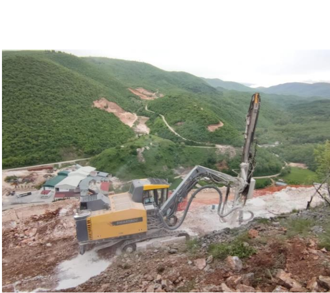
Picture 1: Section 2 service road drilling operation - EW KM7+800
