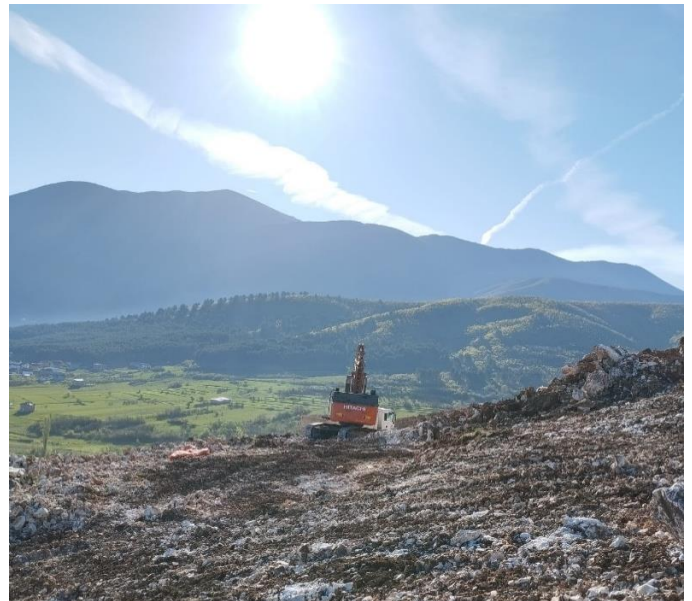
Picture 4: Section 2, topsoil stripping works Km7+450~7+600.
