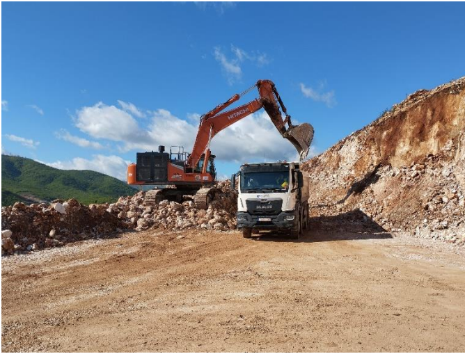
Picture 11: Section 2A Km 7+500 Earthworks Activities
