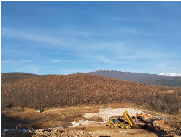
Picture 7: Section 2 - Earthworks
