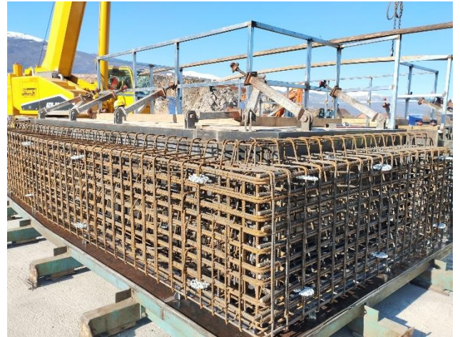
Picture 4: Section 2 - Access Road Rebar Works
