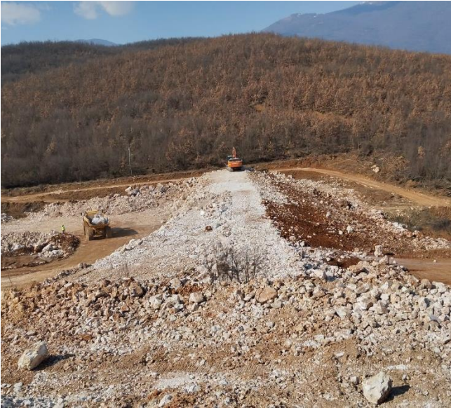
Picture 11: Section 2 - Earthworks
