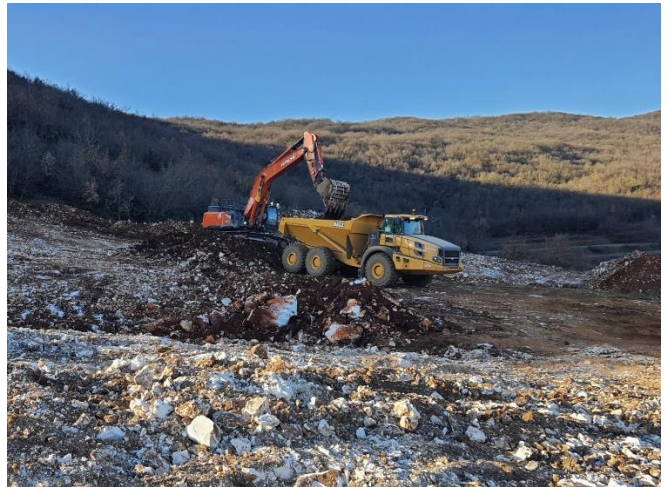
Picture 8: Section 2 - Earthworks
