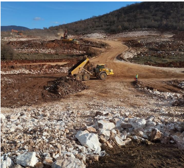
Picture 9: Section 2 - Earthworks
