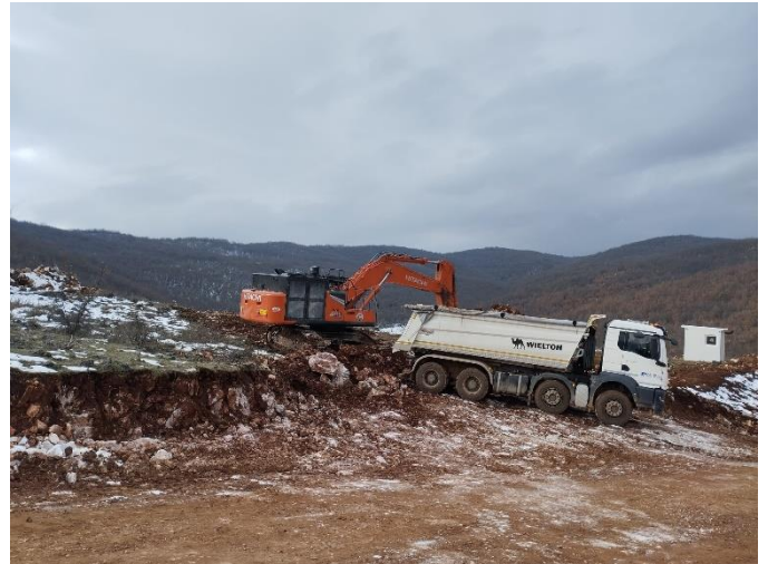
Picture 2: Section 2 - Earthworks
