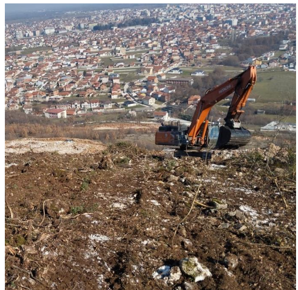
Picture 1: Section 2 - Earthworks
