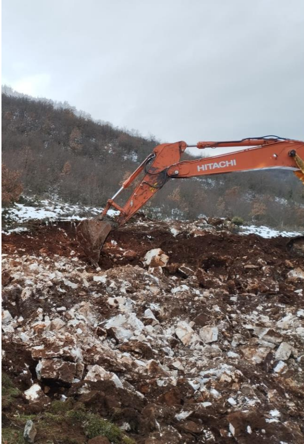
Picture 1: Section 2 - Earthworks
