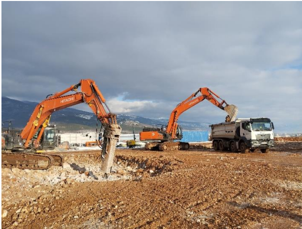
Picture 3: Section 2 - Earthworks
