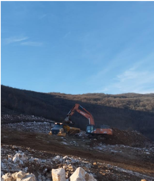
Picture 5: Section 2 - Earthworks
