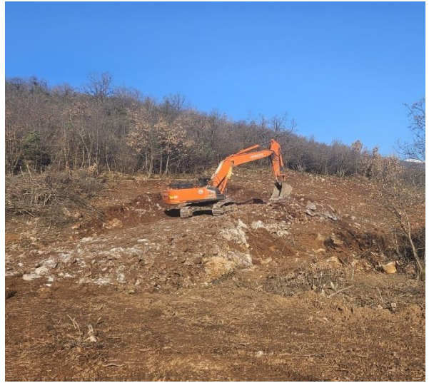
Picture 12: Section 2 - Earthworks
