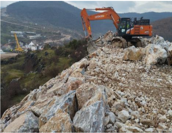
Picture 3: Section 2 - Earthworks
