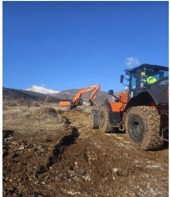
Picture 16: Section 4 - Geotechnical Investigation Work Road
