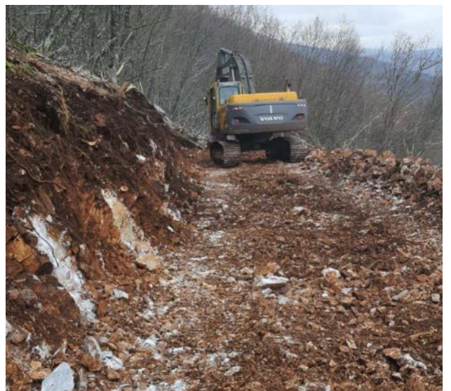
Picture 14: Section 2 - Geotechnical Investigation Work Road
