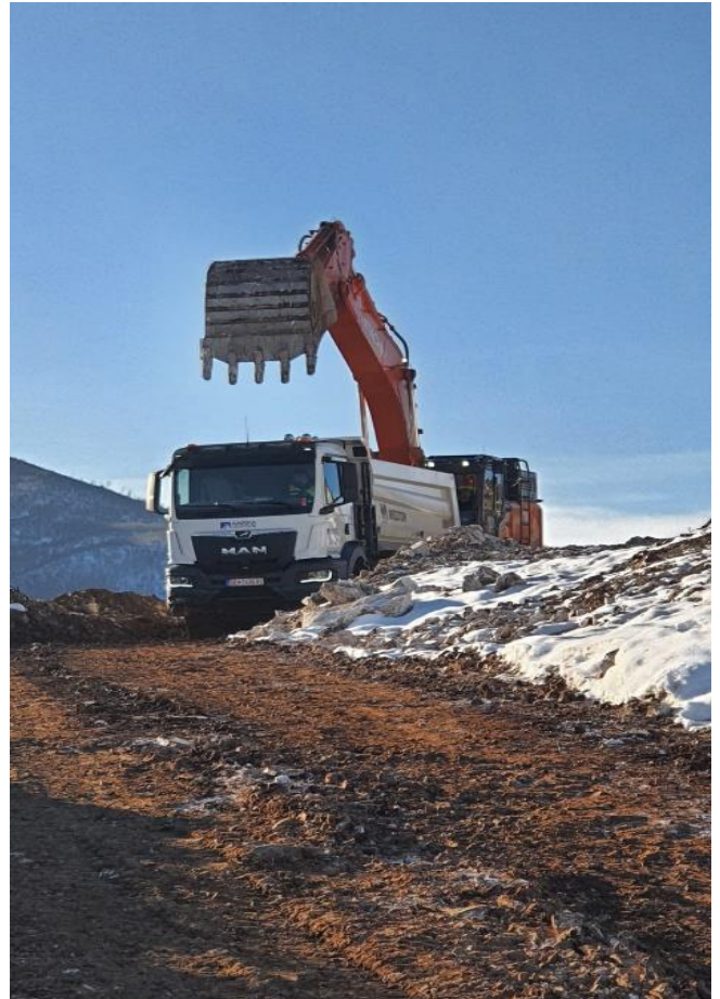
Picture 2: Section 2 - Earthworks
