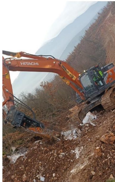
Picture 6: Section 2 - Geotechnical Investigation Work Road
