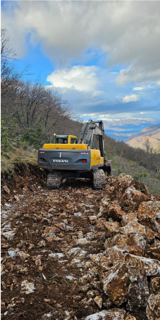
Picture 1: Section 2 – Geotechnical Investigation Work Road
