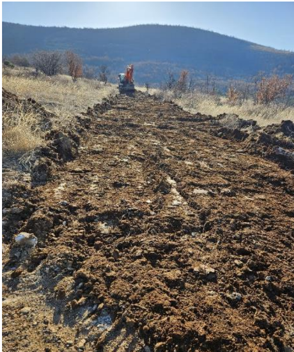
Picture 15: Section 4 - Geotechnical Investigation Work Road
