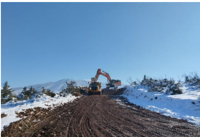
Picture 13: Section 2 – Earthworks
