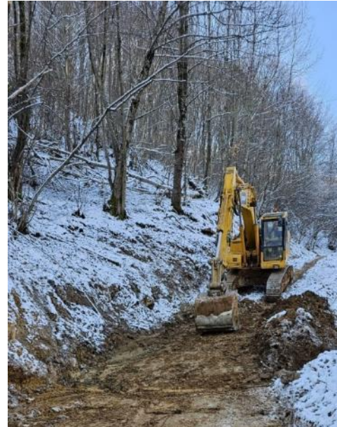
Picture 8: Section 2 - Geotechnical Investigation Work Road
