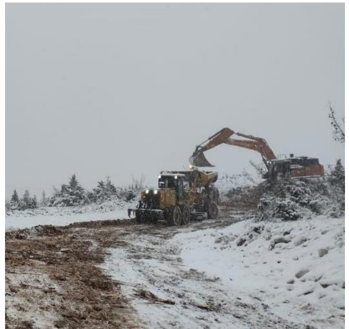
Picture 10: Section 2 - Earthworks
