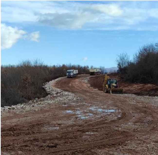
Picture 11: Section 2 - Earthworks
