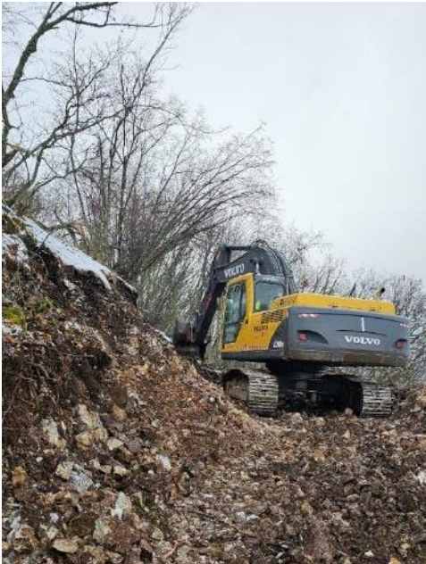
Picture 7: Section 2 - Geotechnical Investigation Work Road
