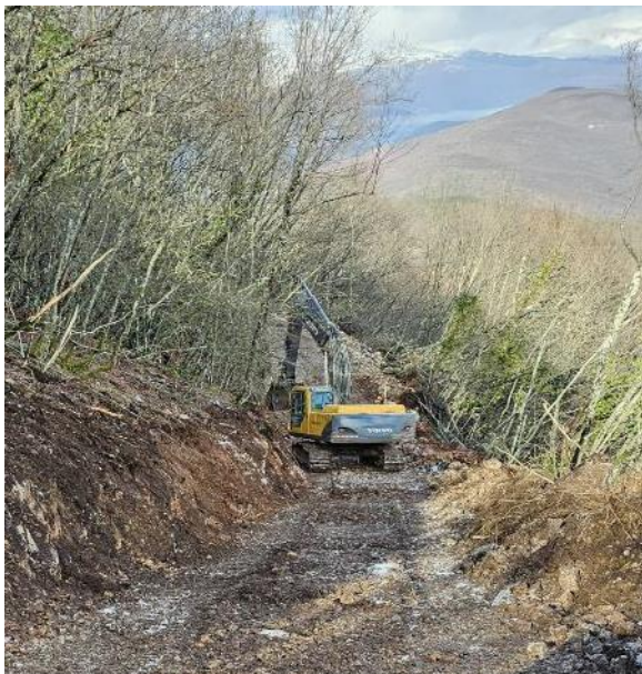
Picture 9: Section 2 –Geotechnical Investigation Work Road
