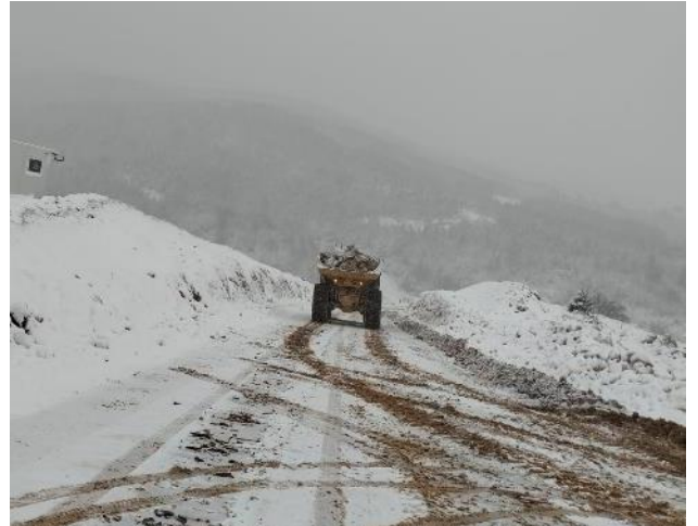
Picture 12: Section 2 - Earthworks
