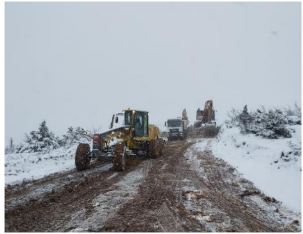
Picture 4: Section 2 - Earthworks
