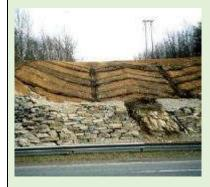
Herringbone and slopes drains are commonly inserted into side slopes to reduce the pore pressures in the slopes. The drains are designed to meet the specific requirements of the slope and its stability. See photograph of drains inserted into an unstable slope.
