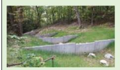
The dams can be constructed from a variety of materials. The example alongside uses concrete but alternative materials such as tree logs or rock filled gabion baskets can also be placed across the stream to form a leaky dam. Rock mounds in the stream bed or rock dams can also be constructed.
