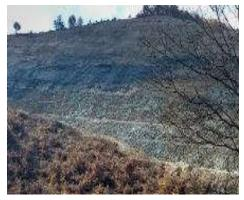
Flatter slopes are more able to sustain vegetation that will assist in stabilising the slope and resisting erosion, and water ingress. The safe angle of repose for a slope will depend on the weakest soil type in the slope.
