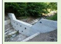
Debris dams are essentially substantial porous check dams. Their purpose is to retain heavy debris brought down a stream within a torrential flow, such as rocks boulders and trees. In normal flows they allow the passage of water through the structure or over the lowered lip. Under torrent flows the boulders etc. are stopped on the upper stream side.
