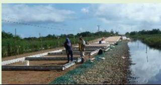
Swale under construction with stone filled mattress protection to embankment visible.
