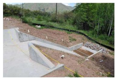
**Reinforced Concrete Spillway to Landslide repair**
