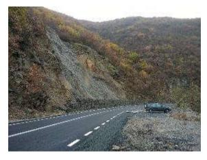
The photograph is an indication of a typical problem for roads in North Macedonia's mountainous terrain where fractured rock results in general rock face spalling, and some larger slippages.
