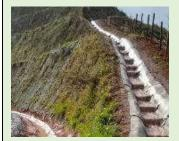
as in the photo. However care must be taken to ensure that any low points in the bench drains profile are designed out or an additional outlet may need to be provided down the slope face.
