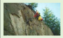
Rope access techniques provide a cost effective and safe means of undertaking scaling work, when carried out properly. All rope access workers should be qualified to the relevant recognised safety standards, for example IRATA (Industrial Rope Access Trade Association) standards or similar.
