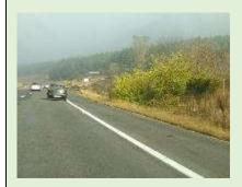
Overedge drainage requires that the road edge is efficiently maintained to remove any build up of debris that can prevent drainage over the edge, and instead, channel an increasing volume of water to a low spot. See example in the photograph alongside taken on the road network. At the low spot excessive water volume will then over flow to erode the embankment slope, and in a short time cut it back to the road edge. The problem is increased where roads are upgraded by widening.
