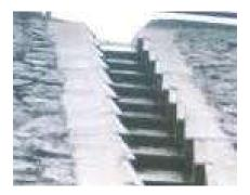
Cascade using stepped precast units
