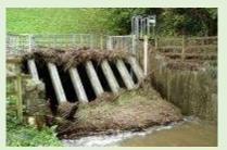
recommended that the screen incorporates has a horizontal section before the culvert inlet to allow for water to pass up and over the screen top and enter the culvert.
