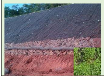
The construction of new slopes can be reinforced by the use of geotextile layers placed on the surface, and nailed into the slope with soil nails.
