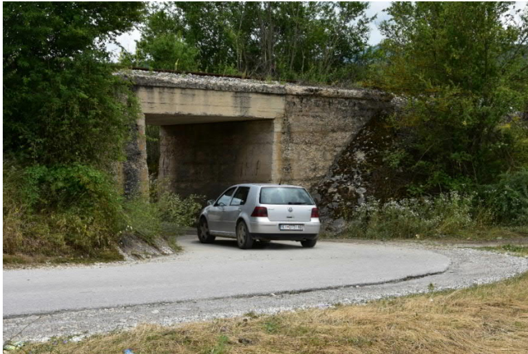
Figure 9-1 - Existing underpass/ box culvert
