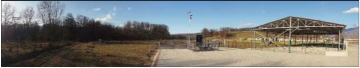
Figure 20-3 – View towards Project Alignment from the small cemetery and mosque in Crvica.
