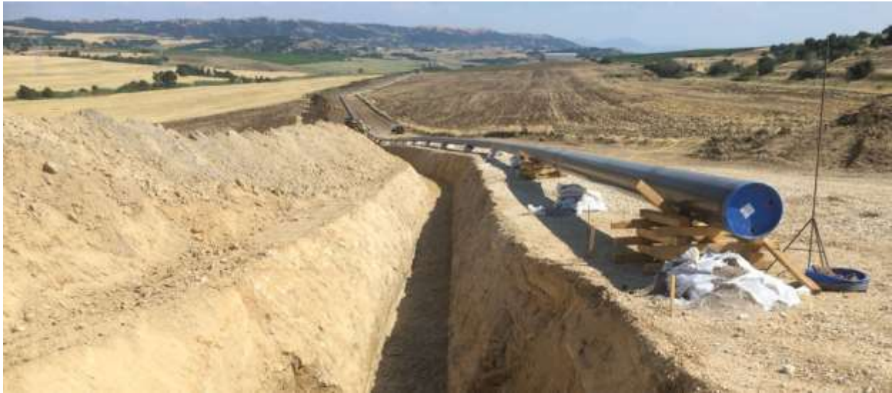
Figure 21.5 – Typical Pipeline Construction
