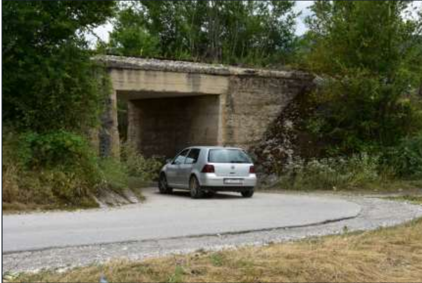
Figure 17-4 - Rail Bridge (at the interchange of “Strogomishte”)
