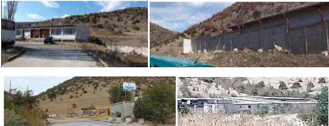
Figure 124 Construction company storage and accommodation facility and a sheep pen
