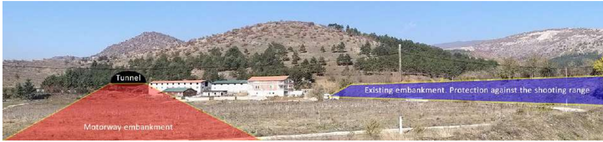
Figure 150 Proposed view of Shooting Range's and Motorway's embankments and the cattle farm
