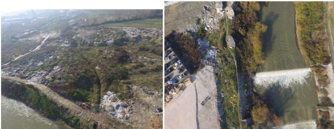
Figure 78 Dumpsite after the railway bridge Figure 79 Dumpsite near the Lepenec' cascades
