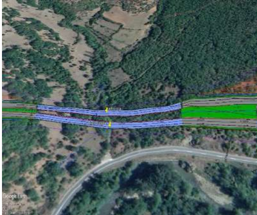
Bridge 1 Left (km 2+145.42 - 2+328.62) and Right (km 2+145.03 - 2+327.10)
