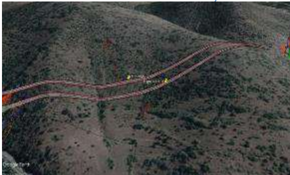
Tunnel 3 Left (km 6+494.90 - 7+499.76) and right (km 6+805.01 – 7+530.00)
