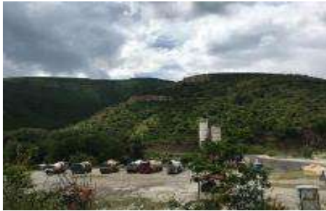
Figure 8 Quarry and separation plant owned by Company Transmet
