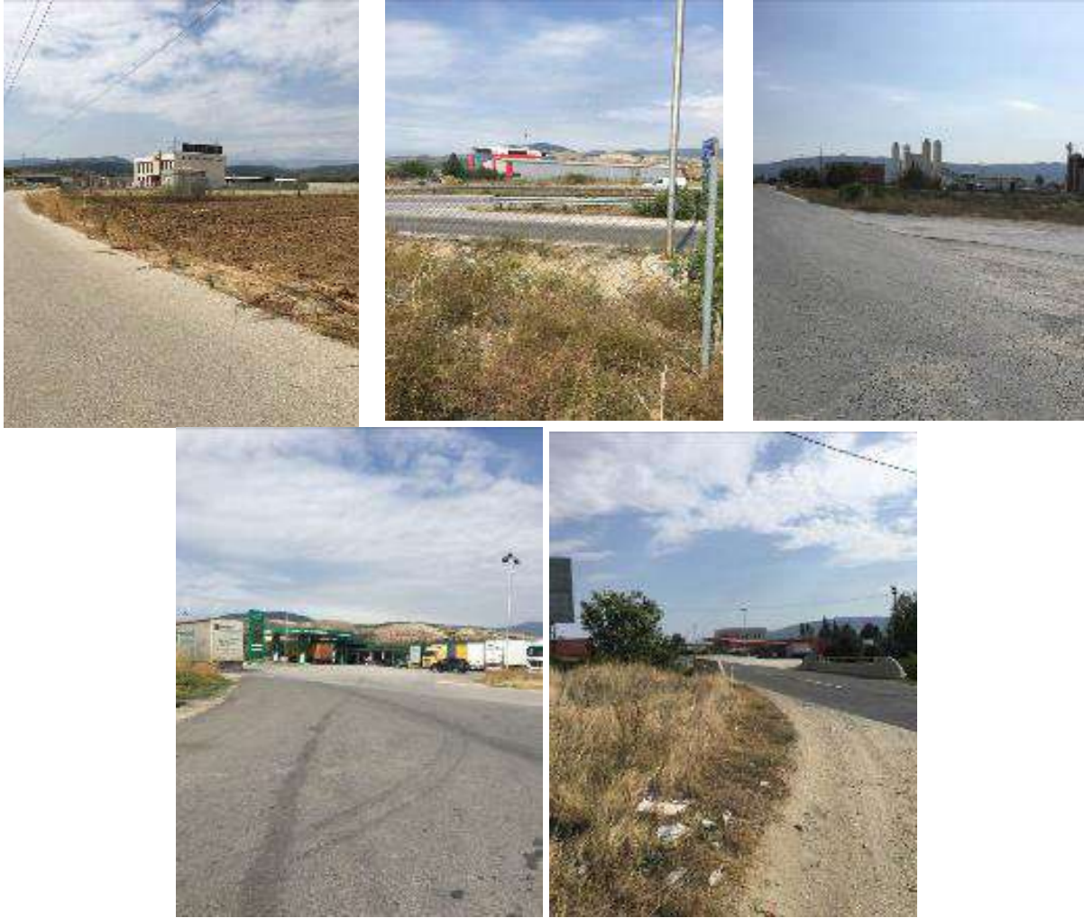
Figure 14 Project area at the south part of the alignment
