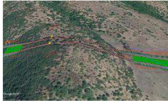
Tunnel 2 Left (km 3+315.79 - 3+596.27) and right (km 3+351.00 – 3+630.00)
