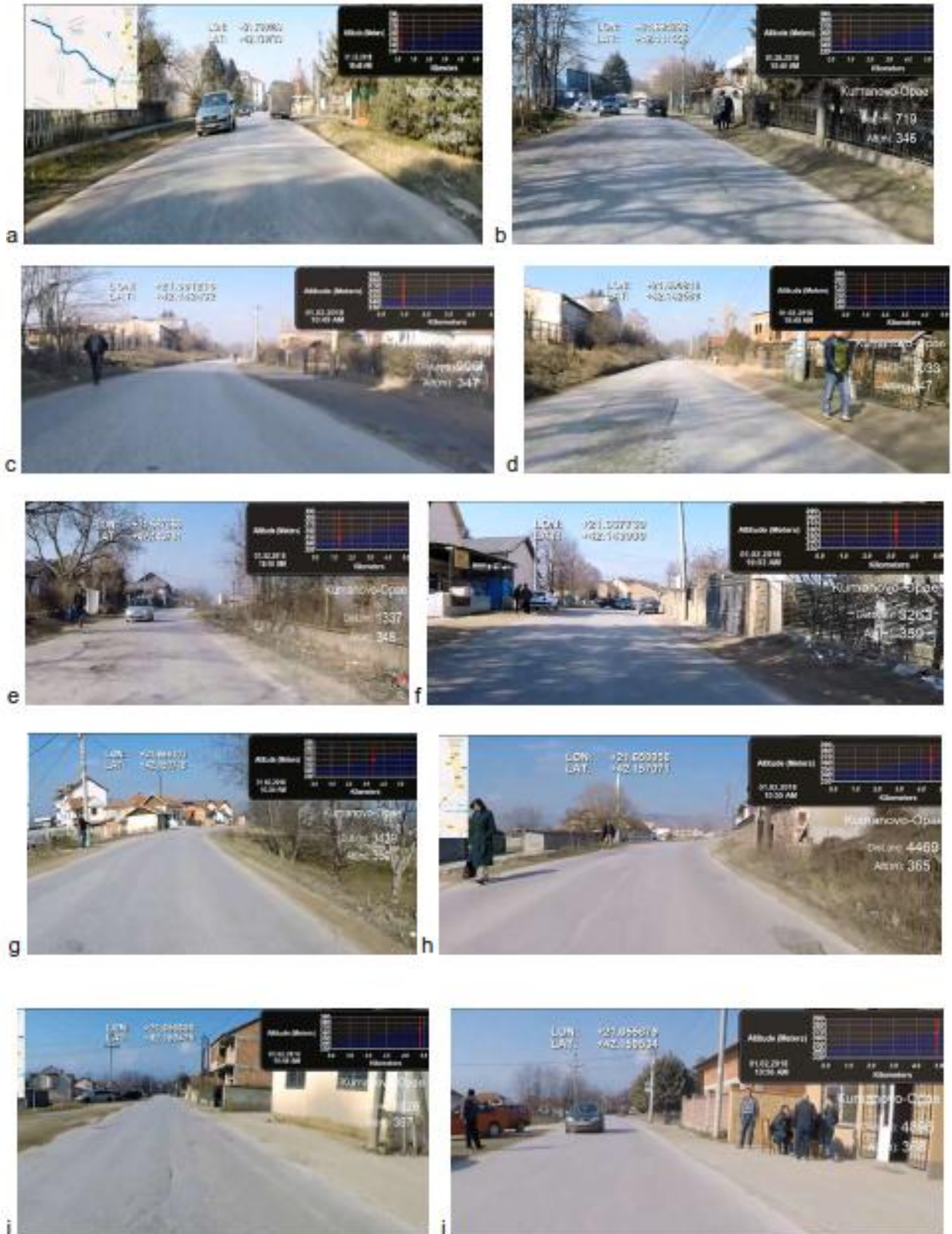
Figure 3 - Photos from the alignment
