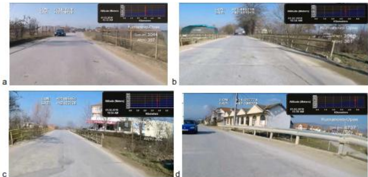
Figure 6 - Photos from the alignment
