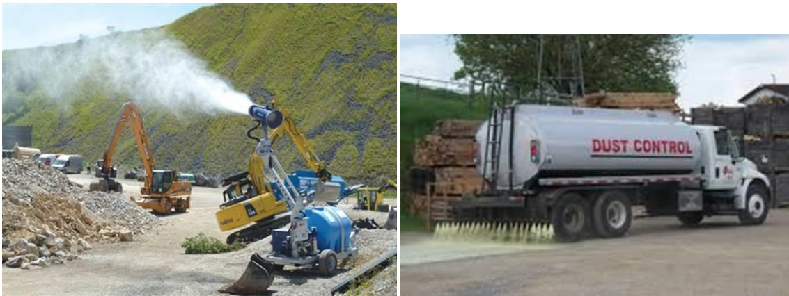
Examples of dust mitigation systems during construction works
