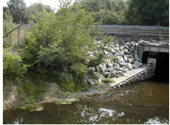
Outline. Bridge (or square section culvert) abutments equipped with tiered river-banks (2 x 0.40 m wide ledges). © BIOTOPE
