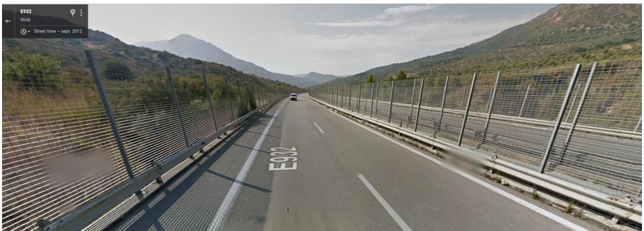
Example of a surrelevated road equipped with a wire mesh palisade to prevent flying fauna from collisions with vehicles
